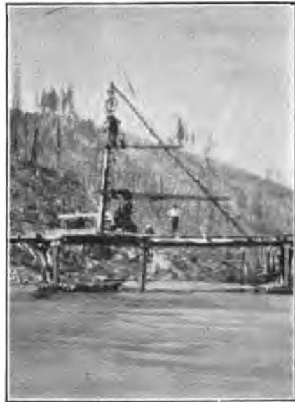
FIG. 11.—Sullivan core drill testing a water power site on the Sugar River, New Hampshire.
